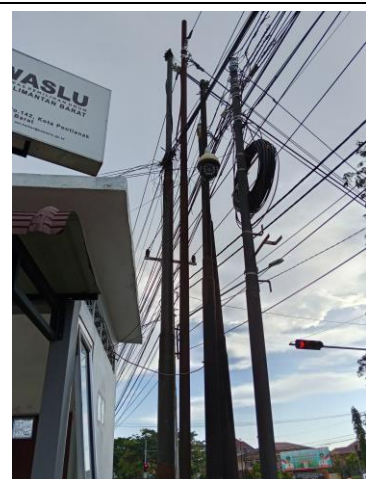
Uraian: Harwat Outdoor Bullet Camera dan Switch Camera (PoE) Outdoor Objek Vital Keterangan: Agustus 2025
