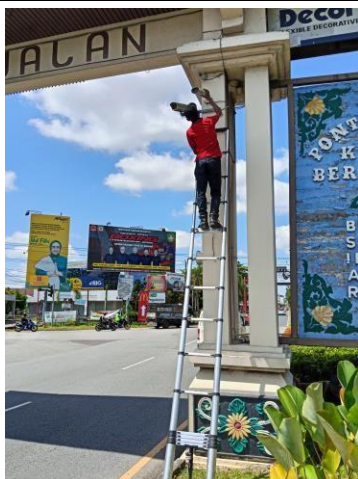
Uraian: Harwat Outdoor Bullet Camera dan Switch Camera PoE Outdoor CCTV Objek Vital Keterangan: Agustus 2025
