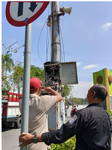
Uraian: Harwat Outdoor PTZ Camera dan Switch Camera PoE Outdoor CCTV Objek Vital Keterangan: September 2025
