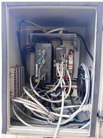
Uraian: Harwat Switch Camera PoE Outdoor CCTV PAM MAKO Keterangan: September 2025
