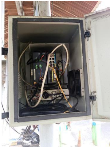
Uraian: Harwat Switch Camera (PoE) Outdoor dan Kabel Jaringan Objek Vital Keterangan: September 2025
