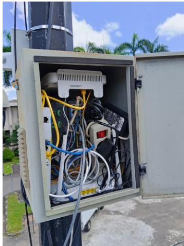
Uraian: Harwat Switch Camera PoE Outdoor CCTV dan Outdoor PTZ camera Objek Vital Keterangan: Agustus 2025
