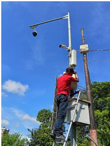
Uraian: Harwat Outdoor PTZ Camera dan Switch Camera PoE Outdoor CCTV Objek Vital Keterangan: Agustus 2025
