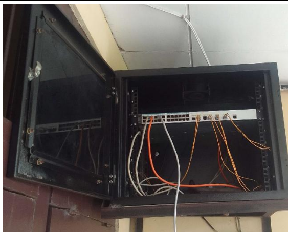
Uraian: Harwat Switch Camera (PoE) Indoor Keterangan: Maret 2025
