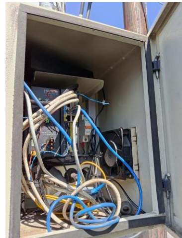
Uraian: Harwat Outdoor PTZ Camera dan Switch Camera PoE Outdoor CCTV Objek Vital Keterangan: Agustus 2025
