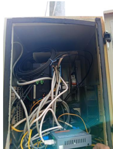
Uraian: Harwat Kabel Jaringan CCTV dan Switch Camera (PoE) Outdoor PAM MAKO Keterangan: September 2025
