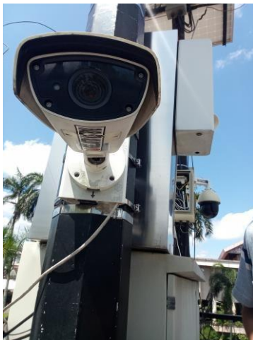
Uraian: Harwat Outdoor Bullet Camera dan Switch Camera (PoE) Outdoor Objek Vital Keterangan: Agustus 2025
