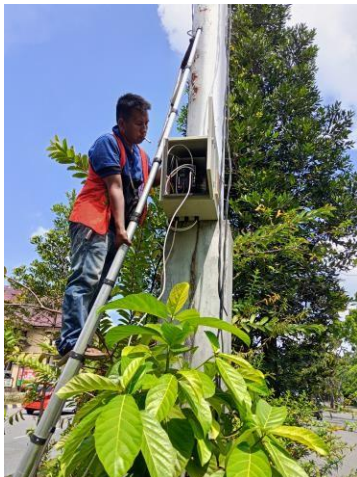
Uraian: Harwat Kabel Jaringan CCTV dan Switch Camera (PoE) Outdoor PAM MAKO Keterangan: September 2025
