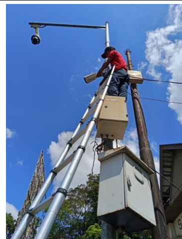
Uraian: Harwat Outdoor Bullet Camera dan Switch Camera PoE Outdoor CCTV Objek Vital Keterangan: Agustus 2025
