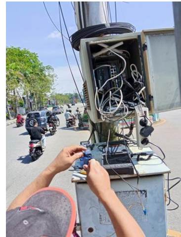
Uraian: Harwat Switch Camera (PoE) Outdoor dan Kabel Jaringan Objek Vital Keterangan: September 2025
